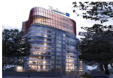
Radisson Blu Hotel & Apartments Douala, Cameroon
